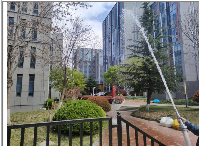
Fire hydrant test
